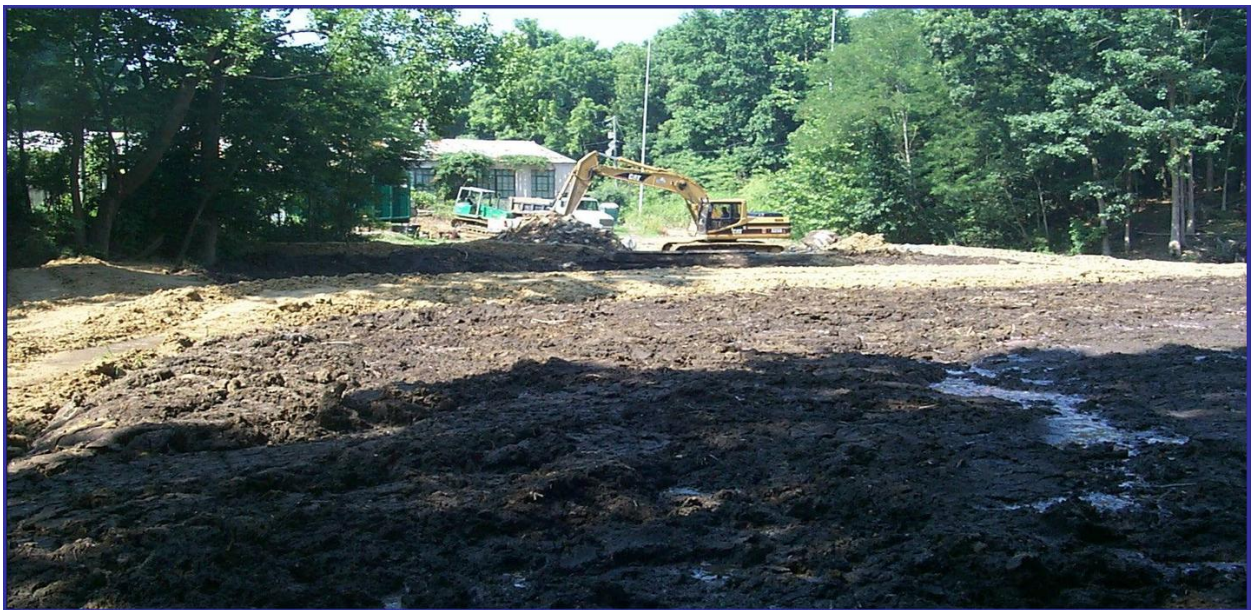
Photo 8. Mixing Adventus amendments into sediments impacted by explosives.
